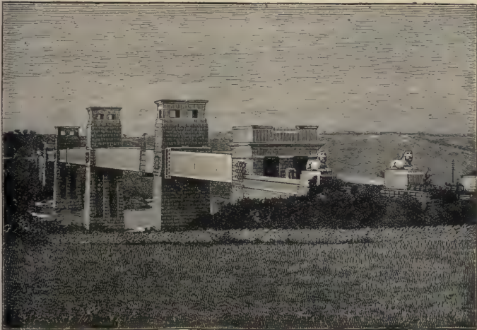
The Britannia Tubular Railway Bridge over the Menai Strait : designed by Robert Stephenson, opened in 1850.
